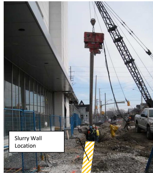
Figure 1. Sheet Pile Installation
