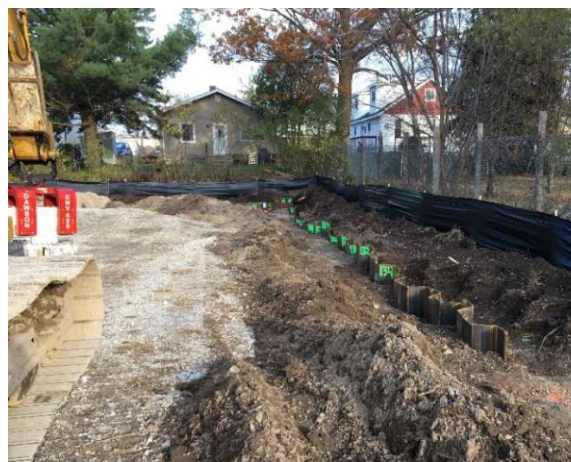
Figure 1 – Property Boundary Cutoff Wall
