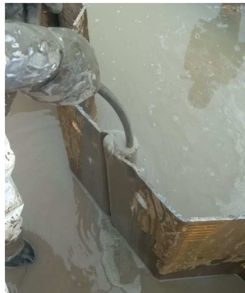
Figure 2 – Grout Tremmie Line
