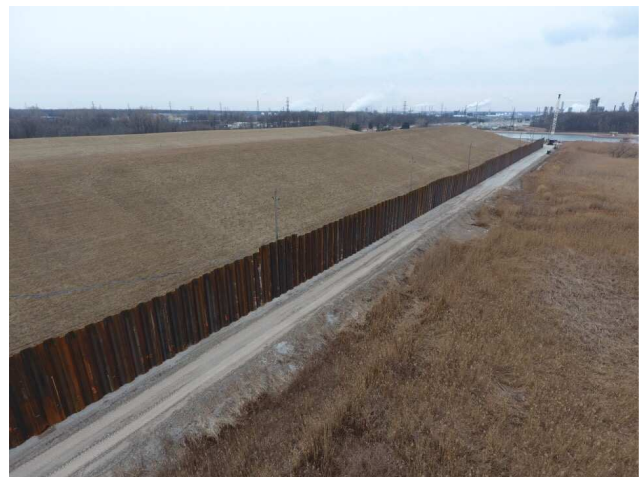
Figure 2. Raked Sheets – North Wall
