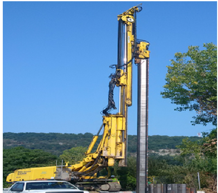
Figure 1. Driving of Sheet pile
