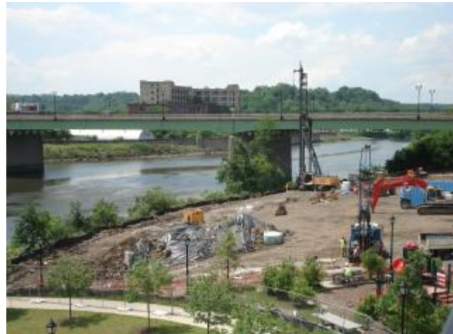
Figure 1. Pile Driving at Former MGP Site
