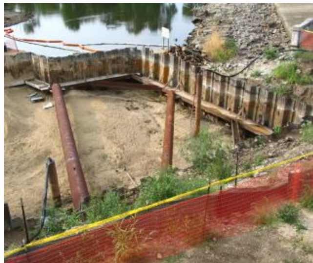
Figure 2. Cofferdam During Excavation
