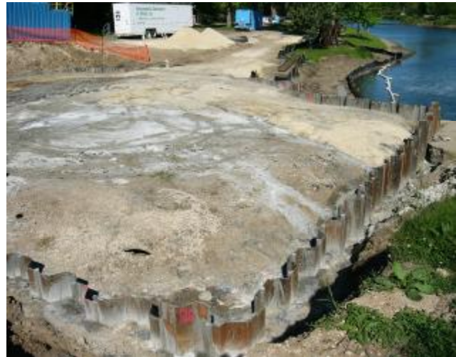
Figure 1. Cofferdam Prior to Excavation
