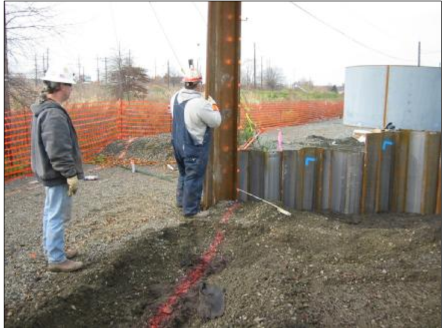
Figure 1: Installation of Custom Bent Sheet
