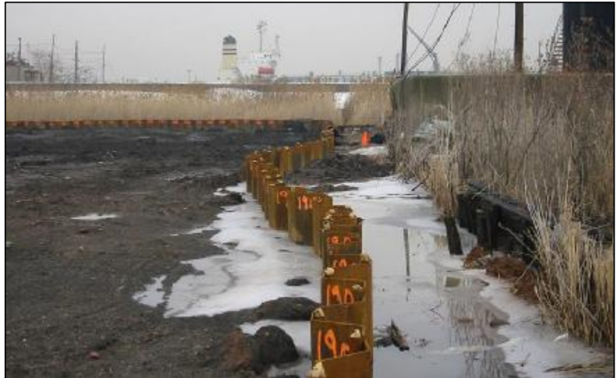
Figure 4: Barrier Along Property Boundary
