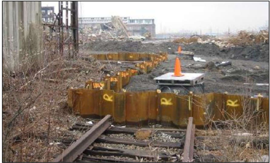
Figure 3: Barrier Through Former Plant
