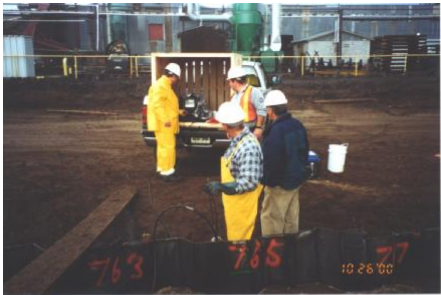
Figure 4: Fibre-Optic Video Inspection
