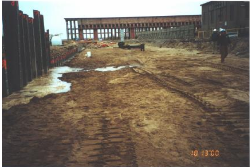
Figure 1: Barrier Along the Pier (Right)
