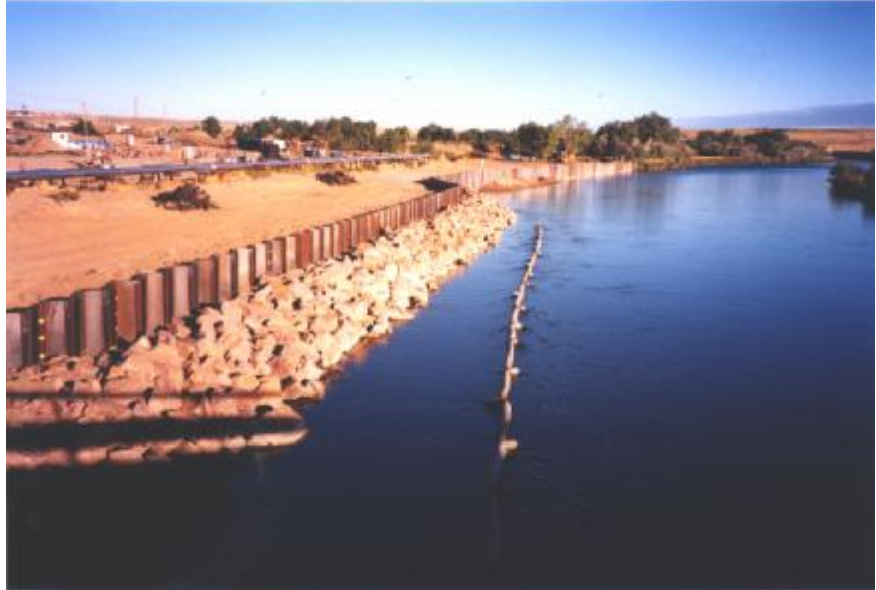
Figure 1: Cutoff Wall and Pump and Treat System
