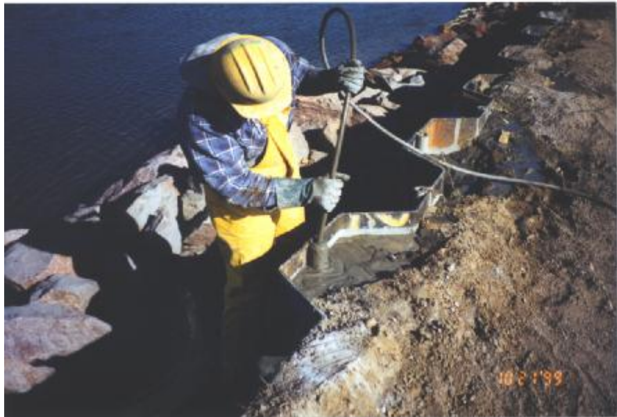
Figure 2: Typical Grout Process
