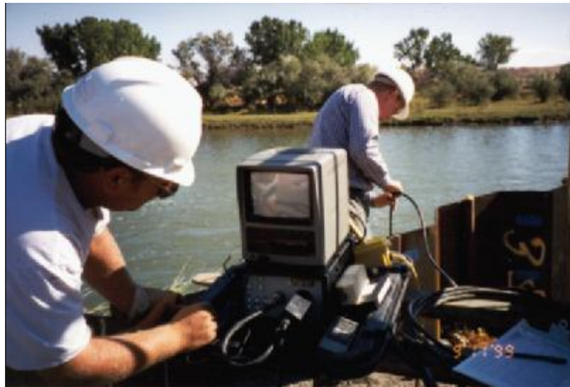
Figure 4: Typical Video Inspection
