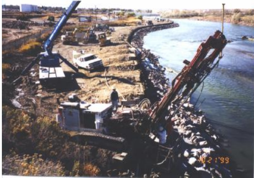
Figure 3: Installation of Tie Rods
