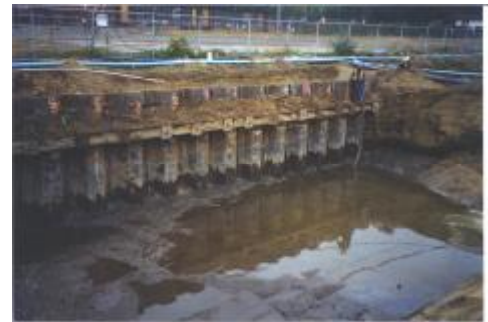
Figure 1. Tie-back Anchor System
