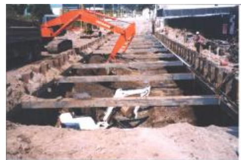
Figure 2. Walers and Struts System
