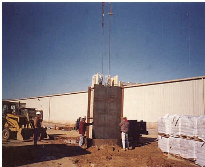
Figure 1. Cassette Installation in Caisson
