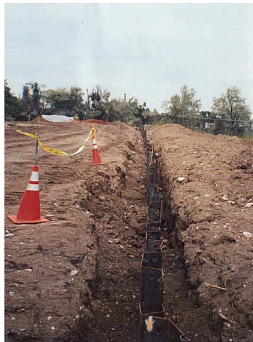
Figure 1. Funnel in Trench
